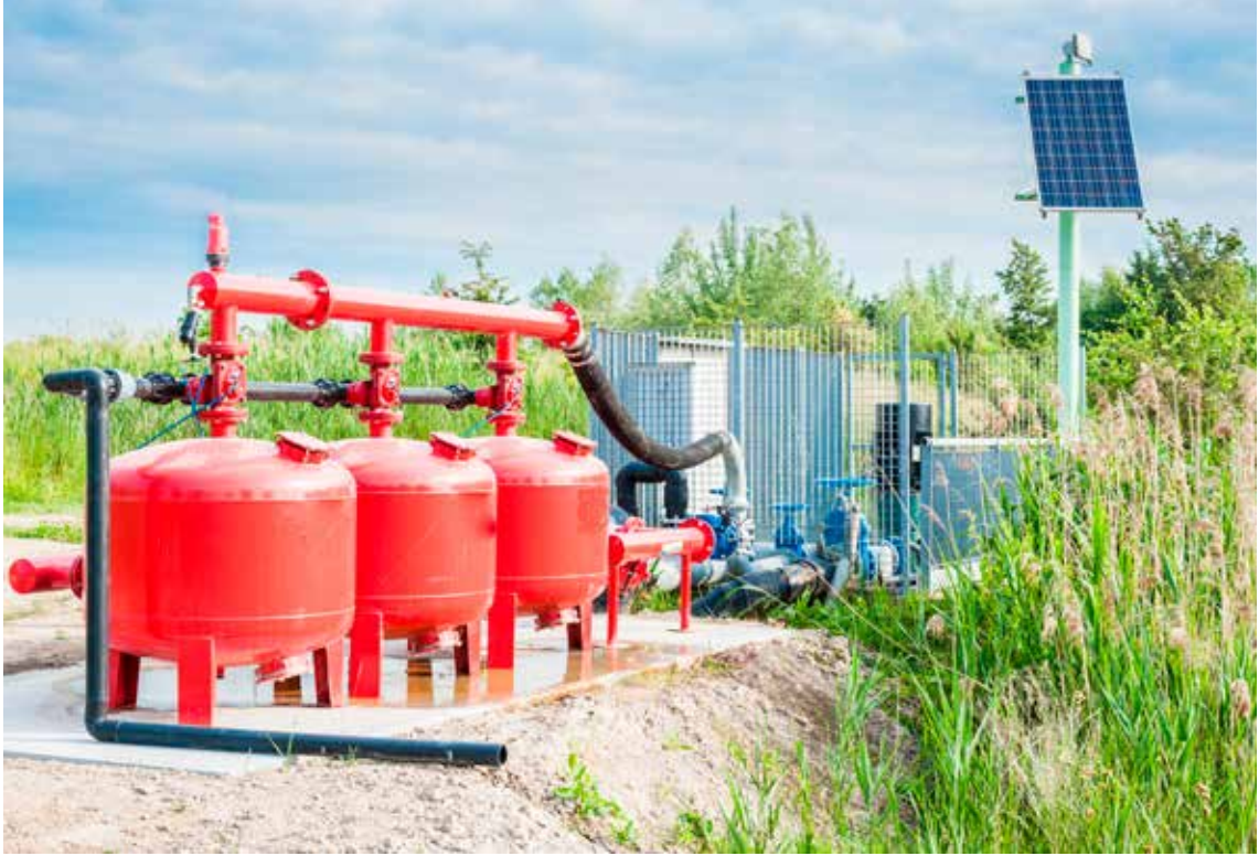
System pumping water for agriculture, with the control unit powered by solar energy © Franco Nadalin - Shutterstock_282434432
