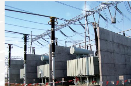
500kV controllable reactor
