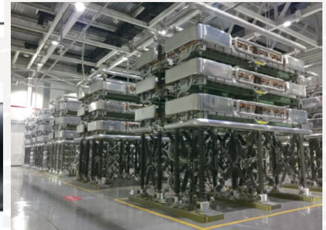
Flexible DC converter valve tower
