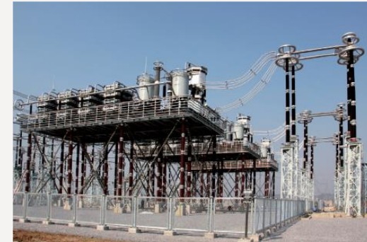
1000kV fixed series capacitor
