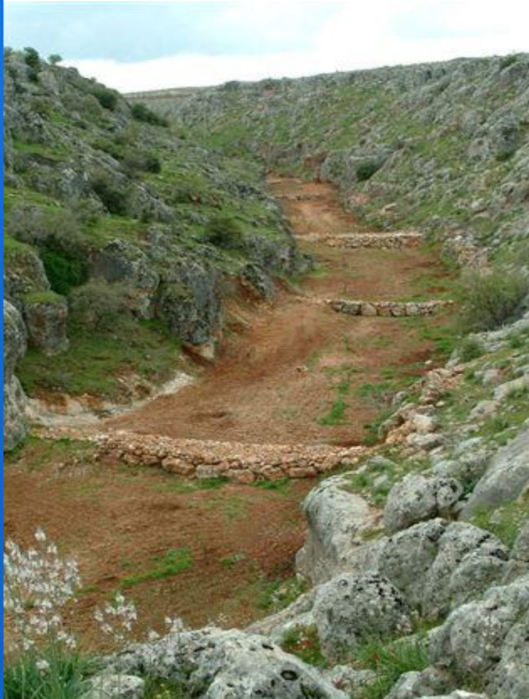
A wadi-bed water harvesting system in Tunisia.
