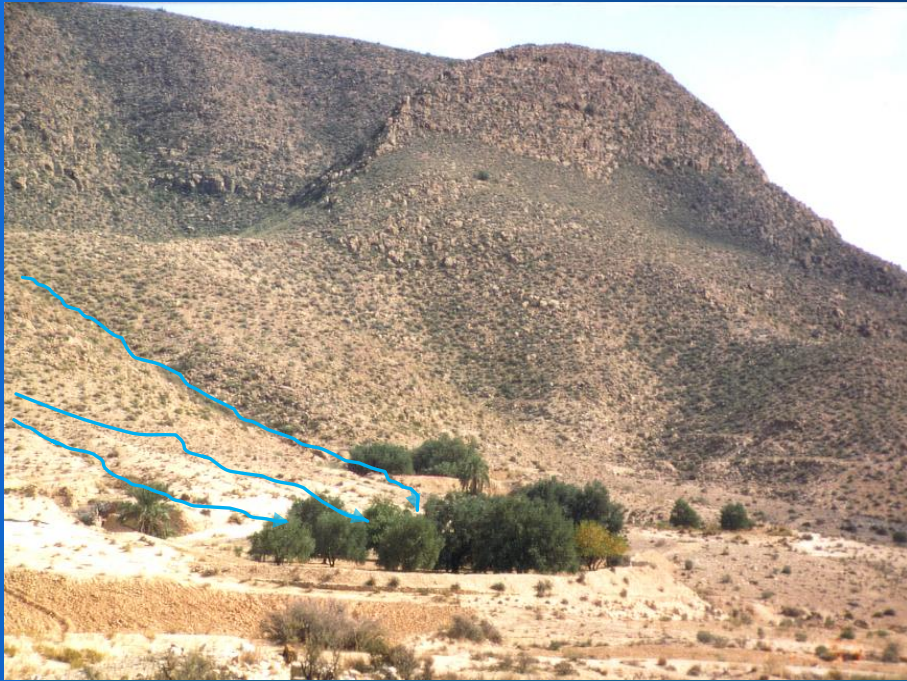
Liman in Tunisia. The bund has a height of about 1.3 m
