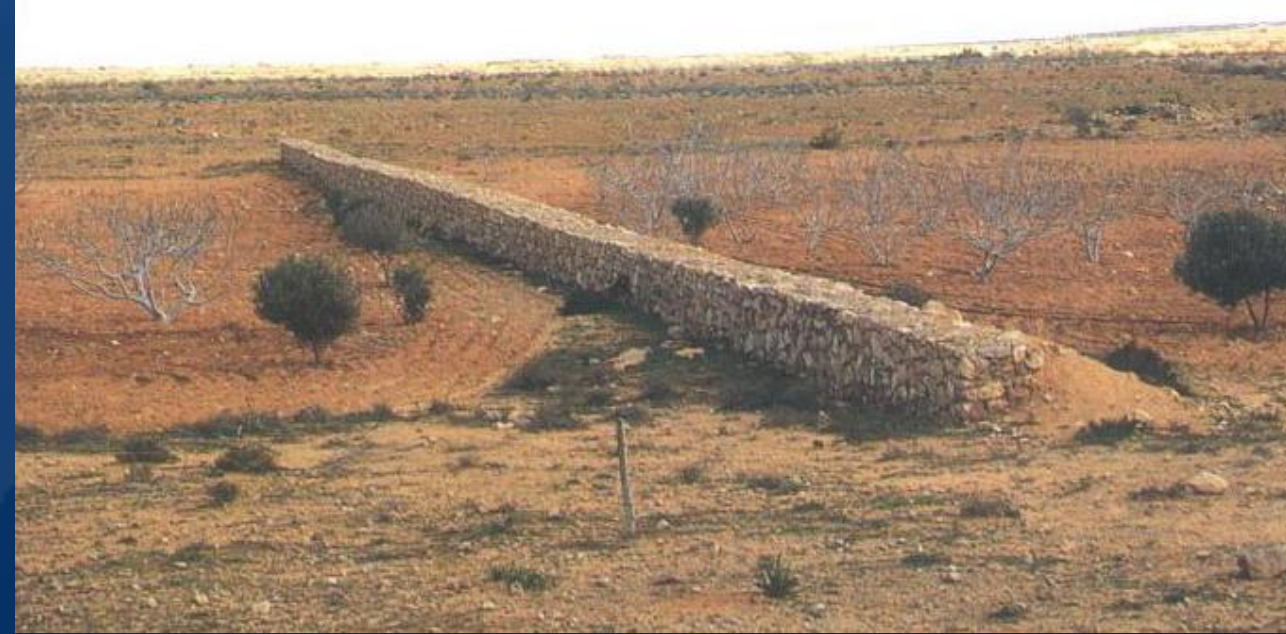
A masonry dam for harvesting floodwater in a wadi in NW Egypt. The water is used for supplemental irrigation of field crops and groundwater recharge..
