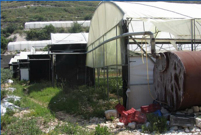
Rainwater tank collecting rain/runoff from greenhouses (Lebanon).
