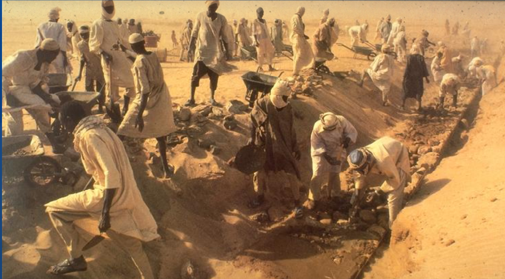
Construction of a groundwater dam in Niger
