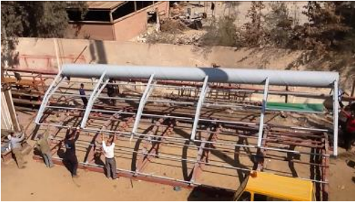
Lifting Trough at shop
