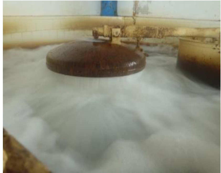
Arrival of the water, dissipation of energy at the load breaker
