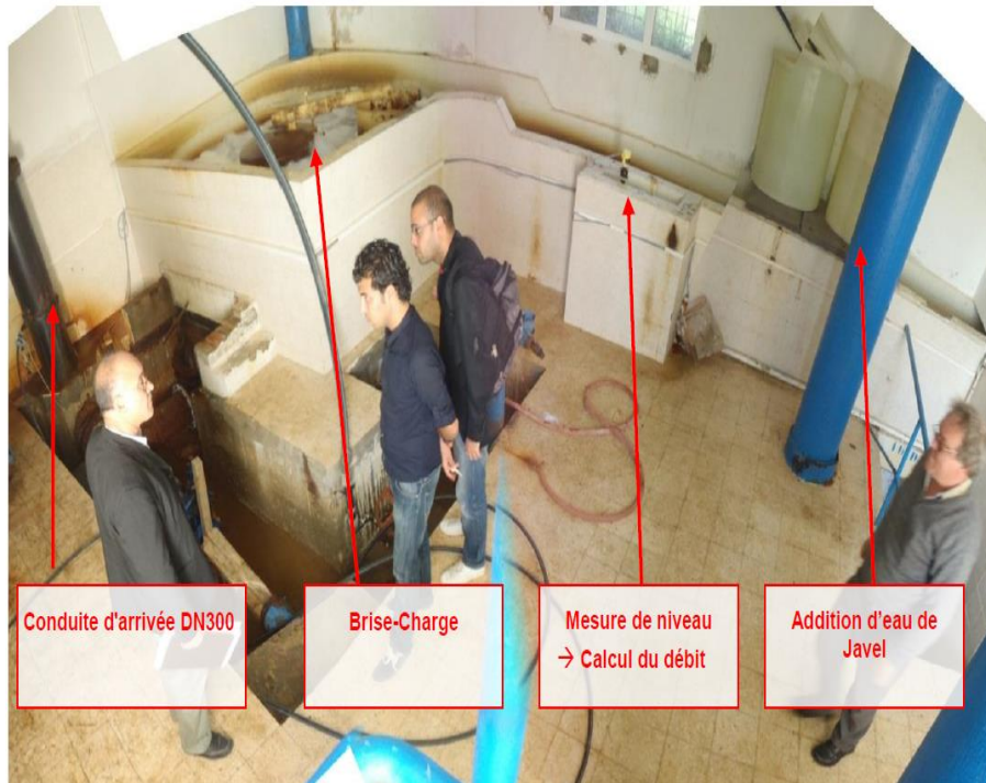
Arrival of the water, dissipation of energy at the load breaker
