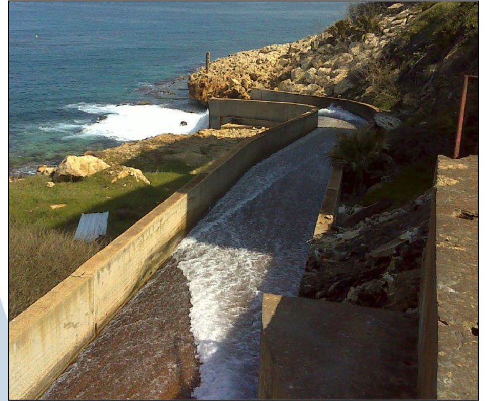
Discharge channels in Zouk and Hreicheh thermal power plants - Source: "Hydropower from Non-River Sources; The potential in LEBANON", UNDP/CEDRO, May 2013
