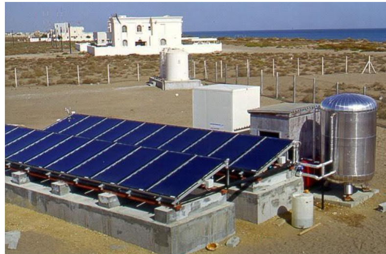
Solar powered desalination plant by Thermosolar in Oman. Photo Credit: Robert Kyriakide's web blog
