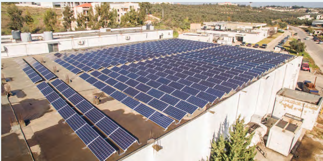
Figure B. Emkan Souk Akkar 120 kWp PV system
